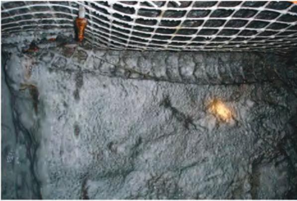
**Figure 3** — Roof and rib 48 hours after gel application.
