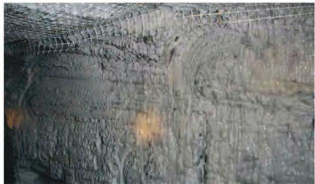
**Figure 2** — Roof and rib after gel application.
