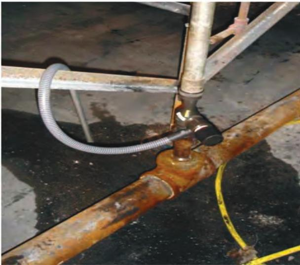
**Figure 4** — Eductor in 1-1/2 in water line.
